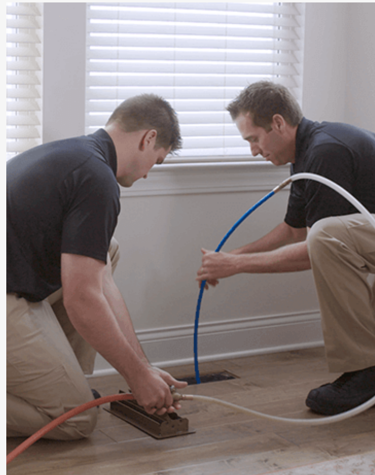
AIR DUCT CLEANING
